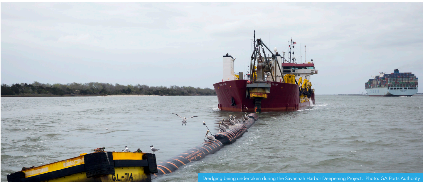
Dredging being undertaken during the Savannah Harbor Deepening Project. Photo: GA Ports Authority
