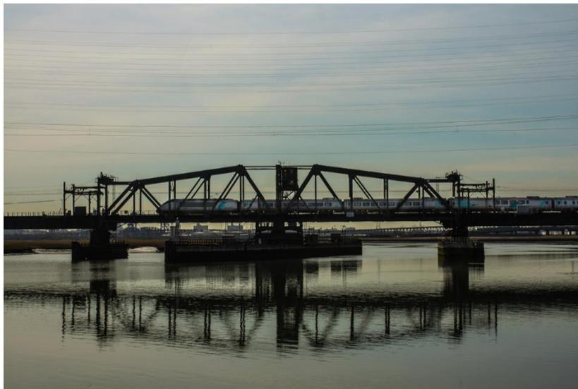
***Portal Bridge is a major chokepoint on the NEC. Completed in 1910, it requires almost continual maintenance, and there are no possible alternative routings to or from New York Penn Station in the event of a failure.***
